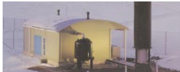
Seutula landfill gas utilisation plant, Vantaa/Finland. Landfill gas, a mix of methane and CO 2 , is explosive and a greenhouse gas of considerable potency. Hence its use for energy has multiple benefits. (Courtesy of Helsinki Metropolitan Area Council YTV, Finland)
