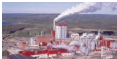
The Enocell Pulp Mill, Uimaharju/Finland, is a modern chemical pulp mill which produces excess heat and power by using process wastes as fuel. (Courtesy of Enso Group, Finland)
